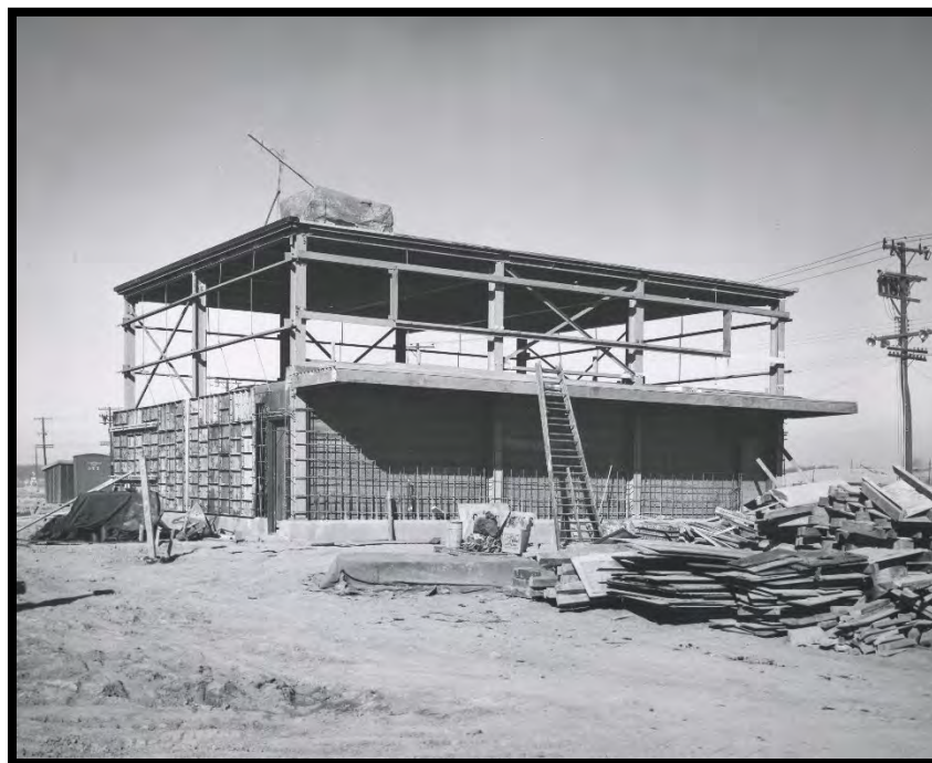
Figure 9: Steel Framework for the X-342B Fluorine Storage Building, April 1954
