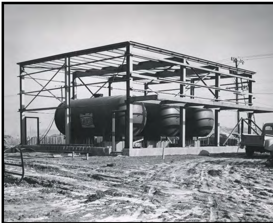
Figure 8: Steel Framework for the X-342B Fluorine Storage Building, February 1954
